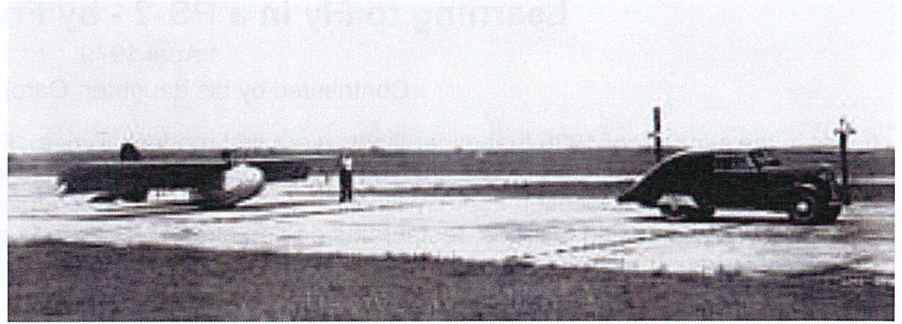
Franklin PS-2 training glider is about to be towed aloft by the specially modified car in front.
