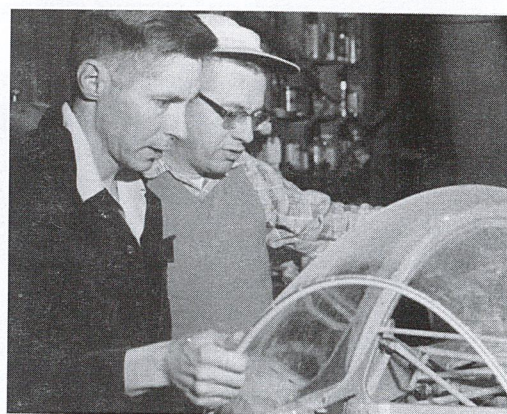
Leonard Niemi (left) and George Coder work on fitting the prototype Sisu canopy. Terry White, NSM Archive.
