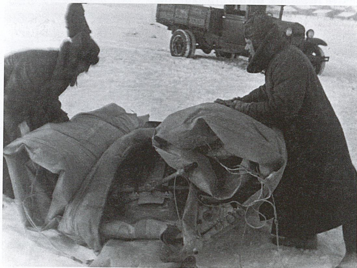
Left, the Grokhovsky rubber glider; Right, folding up the deflated glider after a test flight. NSM Archive.
