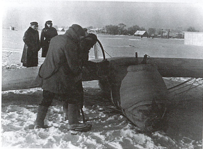
Left, the Grokhovsky rubber glider; Right, folding up the deflated glider after a test flight. NSM Archive.
