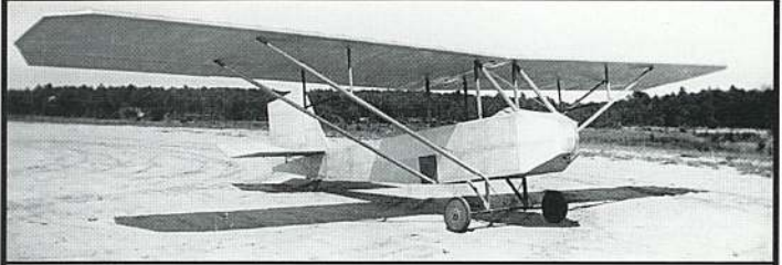
Single place glider CAA #11544, designed and built by Sanders V. Hudson Jr. at E. Durham, NC, "minus a single braze or rivet, using only bolts and clamps," January to Aug. 10, 1932. Flew 700+ flights - Rebuilt in Spring 1934 into a motorglider.
