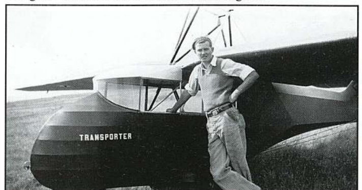
Jay Buxton's two-place "Transporter" sailplane after addition of a 35 hp engine - top speed 65 mph. 1934, California (NSM Multi-Media Archives)
