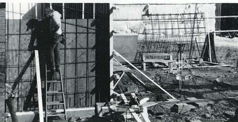
Foundation work during the second & third weeks of August.
