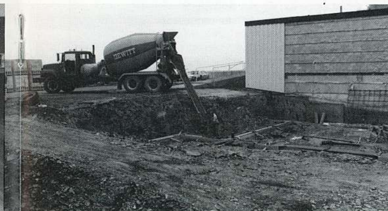
Excavation, during the first week in August.
