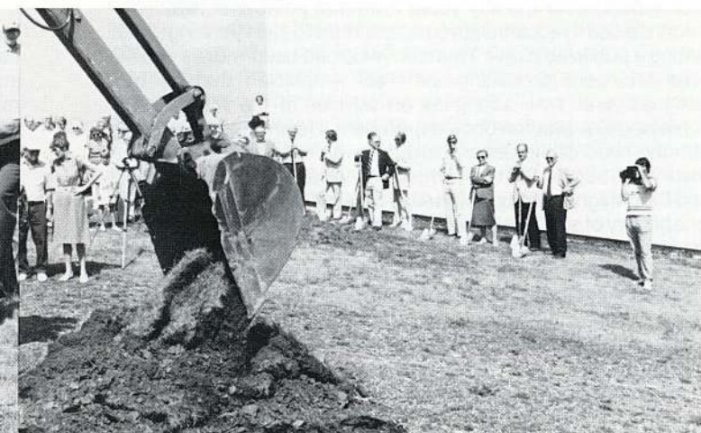
... Then the husky backhoe takes over ...
