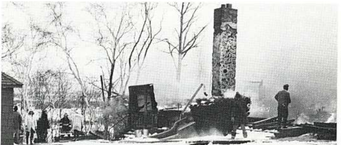
The totally destroyed Harris Hill Administration Building after the January 1977 fire.
