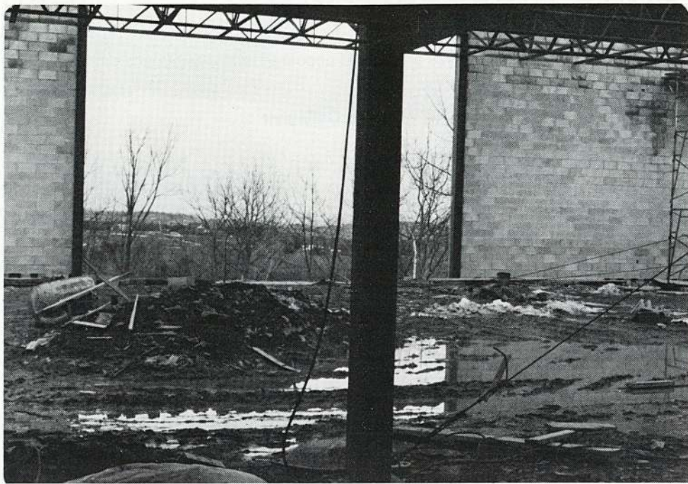
Rear, lower level view of the main Exhibit Hall. March 1978.
