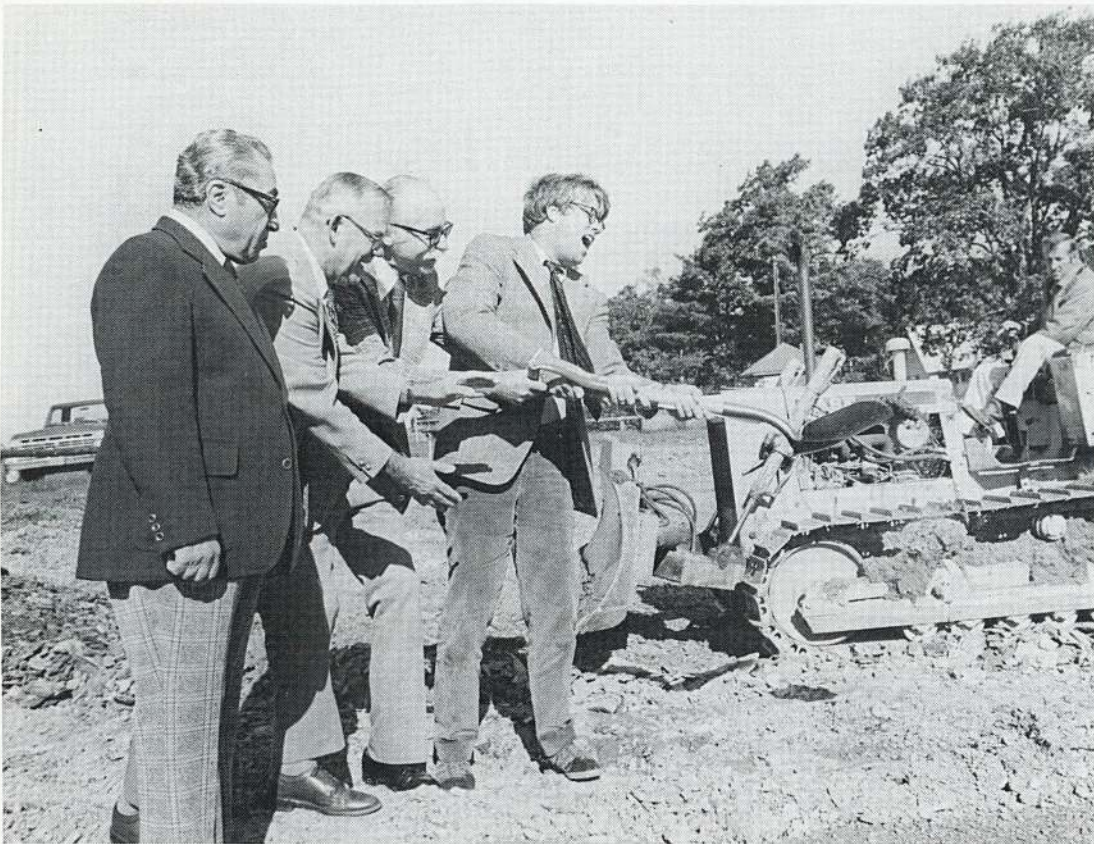
First shovels of earth. (From left) Peter Chalk, Chemung County legislator, Paul Schweizer, SSA director and museum trustee, Bernald Smith, museum president, and William English, museum director, lifted the symbolic first shovel of earth, while a bulldozer waited to do the big job.
