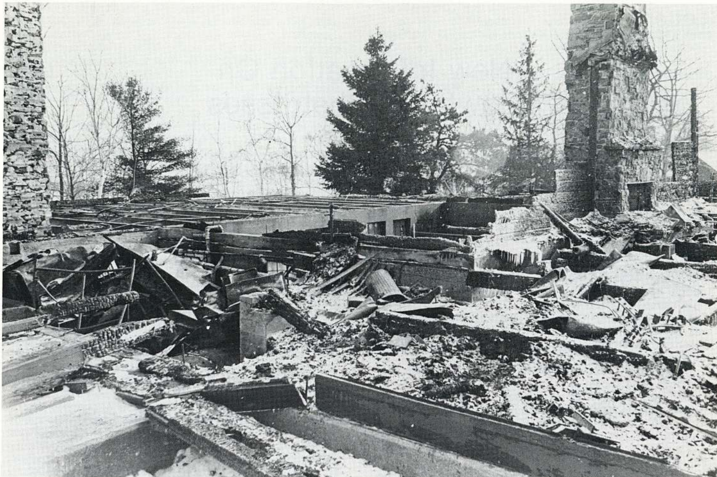
The next morning: Devastation after the Administration Building fire. The chimneys have since been knocked down
