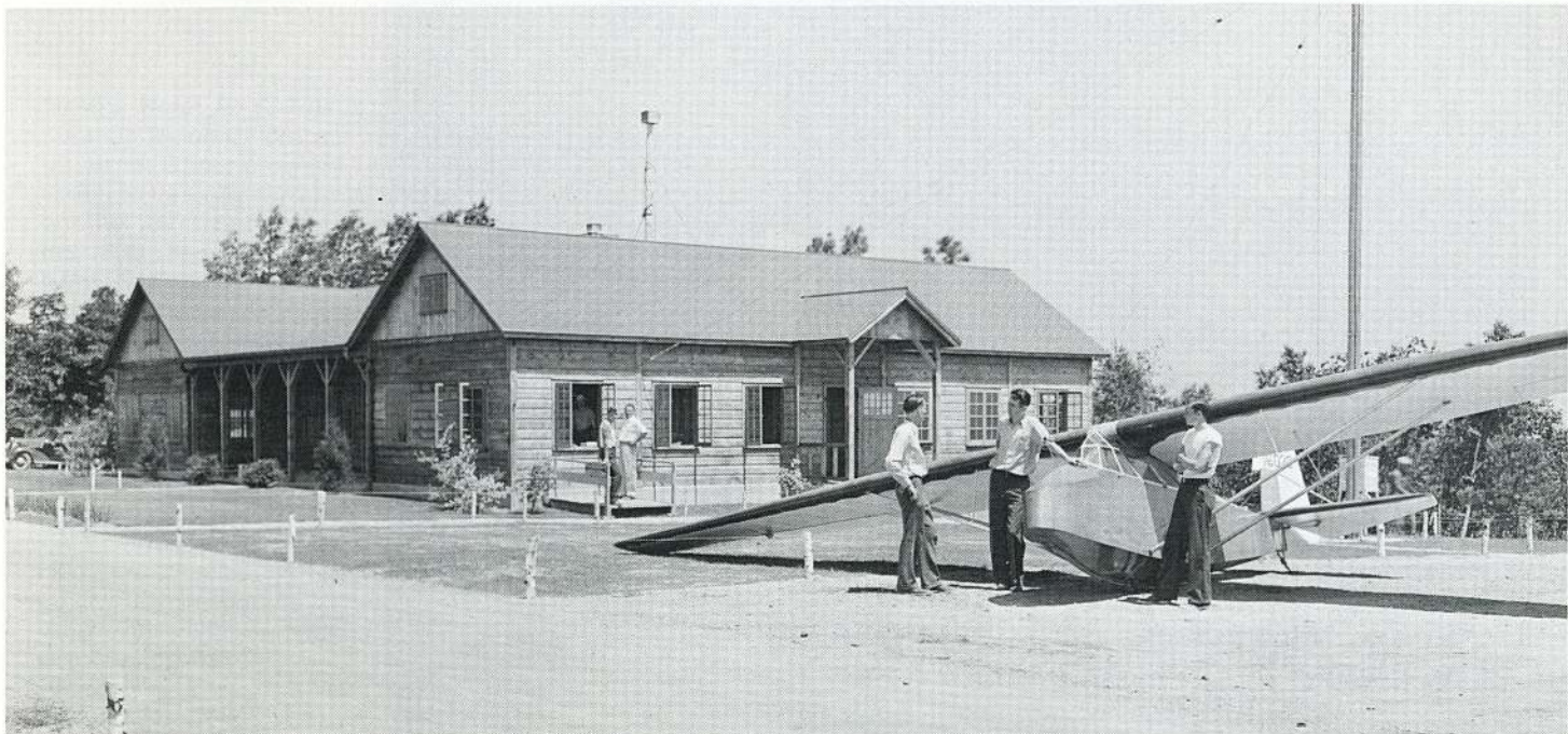
In the beginning: Dedicated in 1937, the Administration Building was closely tied with soaring from the first. It served
